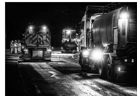
Richard Prior, United Kingdom, Roadworks
